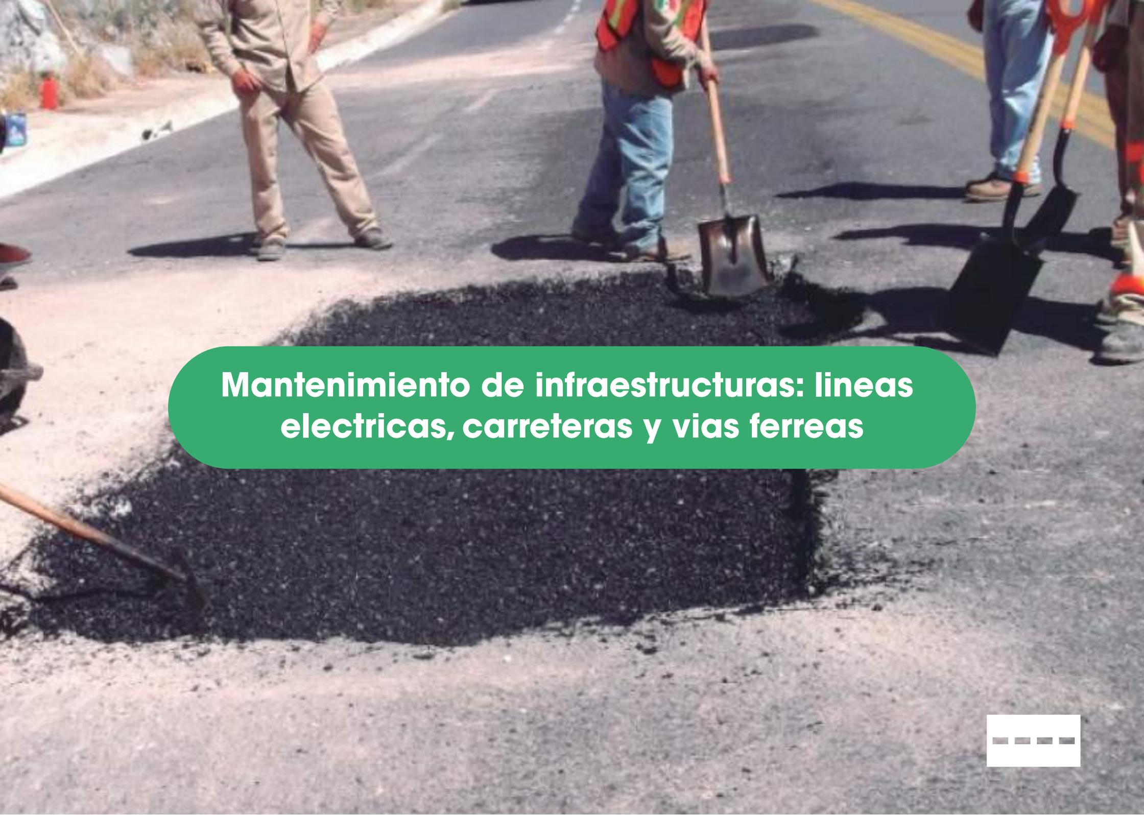
A photograph showing several construction workers on a road. One worker in the center is using a shovel to spread a thick layer of dark asphalt. Other workers are visible in the background, some standing and some using tools. The scene is outdoors on a bright day, with shadows cast on the road surface.
